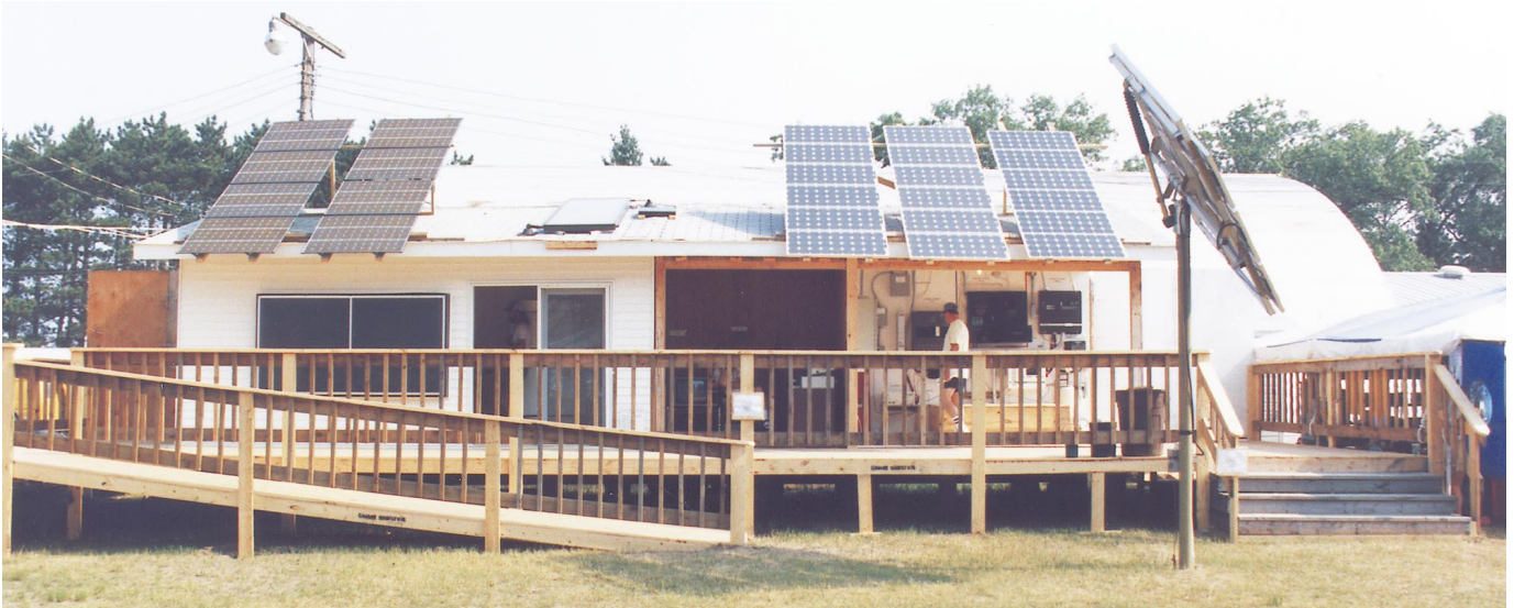
Above: This model home demonstrates wind and photovoltaic electricity, efficient insulation, solar water heating, a low water-consuming bathroom, and the latest in super-efficient home appliances. I had to shoot this early Sunday morning because the booth was too crowded with people when the fair was open to the public.
